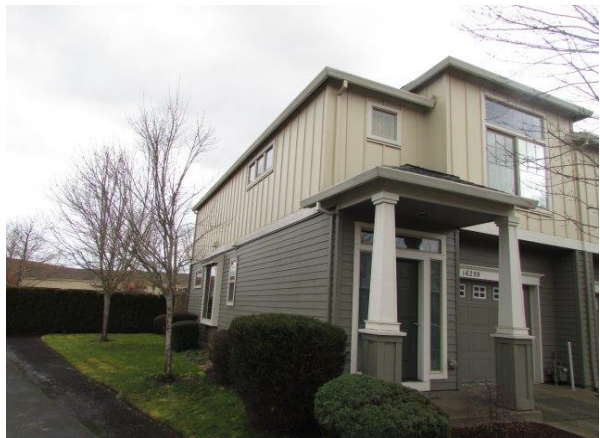
Siding & Trim Repair
