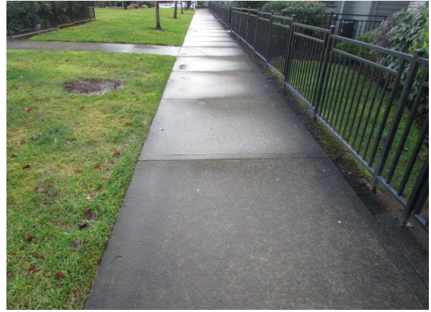
Concrete Safety Repair
